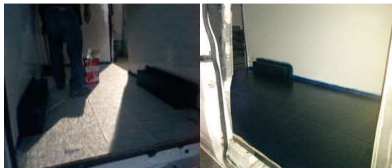
Figure 6. Placement and painting of the fiber
